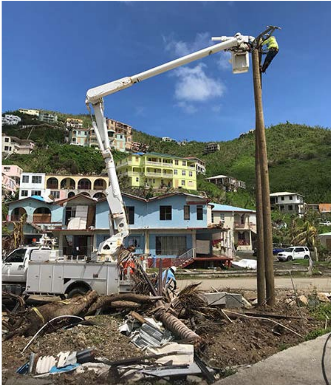
A CUC lineperson assists with attaching pole line hardware to a newly planted pole on Tortola, British Virgin Islands.
