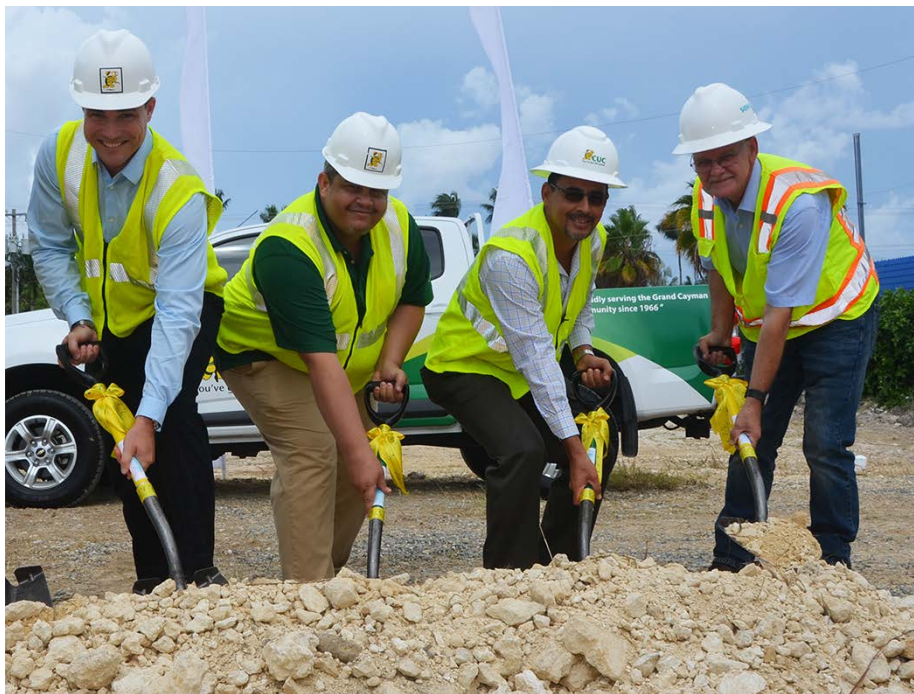
CUC officials (from left) Sacha Tibbetts, Jason Burke and Richard Hew and Hans Czeslik from Siemens, participating in the groundbreaking event.
