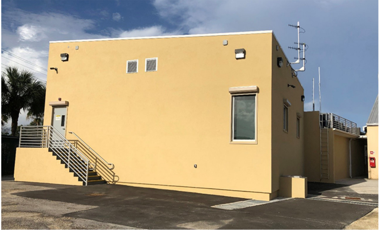
CUC's Technology Building that houses the Company's new Control Room
