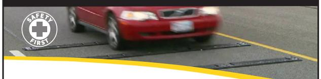
In an effort to alert approaching drivers of speed restrictions when entering an area of road where CUC vehicles and personnel are present, the Company deploys Rumble Strips. These Rumble Strips are a series of raised transverse rubber strips laid across the road, which changes the noise a vehicle's tyres make on the surface and so warning drivers of speed restrictions.
