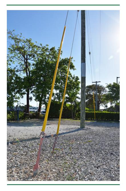
Do not loosen or come into contact with the guy wires or guy rods at the base of poles. These guy wires and rods are marked with a yellow plastic covering. Damage to these wires and rods can result in service interruptions or injuries to the public.
