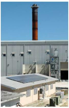
5.4 kiloWatt solar panels (photovoltaic) were installed on the roof of a North Sound Power Plant generation site building.
