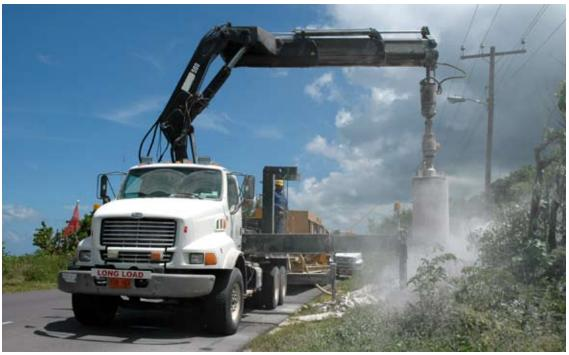
Work continues on the 69 kV loop linking the eastern end of Grand Cayman, which will improve reliability to customers in the districts of North Side and East End. To date, over 200 concrete poles have been installed. Completion of the 69 kV line is anticipated for late 2009 and energising the line is scheduled for early 2010.
