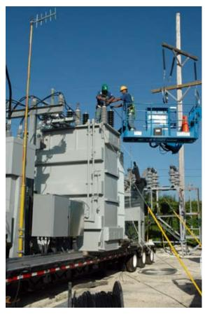
A mobile substation was assembled, constructed, installed, tested and commissioned in 2008 by members of the Company's Electrical Maintenance and Engineering Departments. The mobile substation was installed at the South Sound Substation to substitute for one of the transformers, which was shipped to the United States for repairs.
