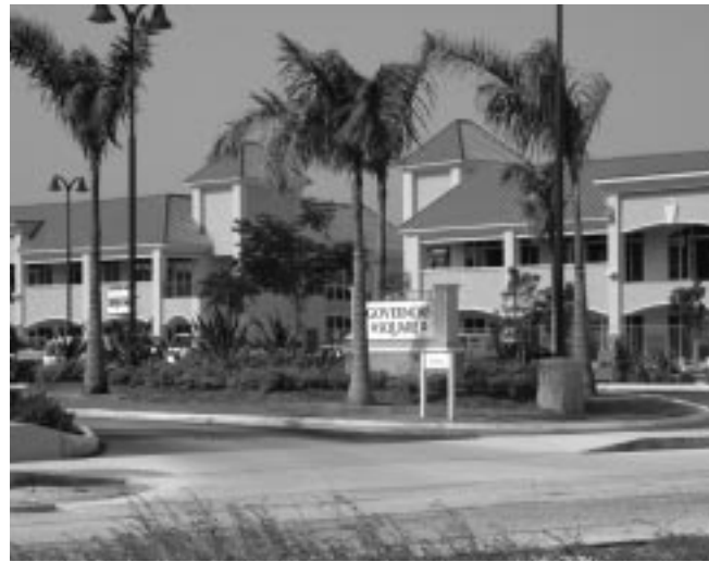
Commercial electricity sales increased 9% as compared to first quarter fiscal 2007 primarily because of new developments such as the 160,000 square-foot Governor's Square shopping and office centre located on West Bay Road.
