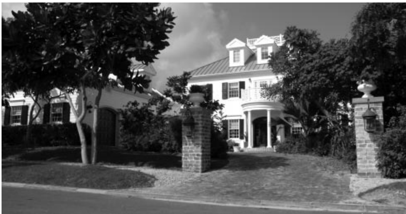
Residential electricity sales increased 8% compared to first quarter fiscal 2007 primarily because of newly constructed high-end residential communities such as Cypress Pointe and Salt Creek (above) on West Bay Road. CUC expects to add 1,800 new customers during fiscal 2008.
