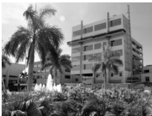
The seven-storey Butterfield Bank building, located in central George Town, is scheduled for completion in July 2007.
