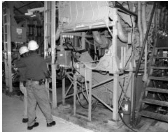
The hurricane-damaged Caterpillar units were repaired and came online in June 2006.
