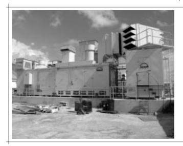
The newly installed 8.4 MW gas turbine is scheduled for commissioning in August 2006.
