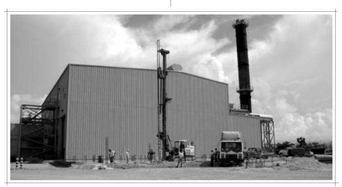
Expansion of Engine Room 5 has commenced to accommodate the new 16 MW V48/60 medium speed diesel generating unit. The unit is scheduled for commissioning in summer 2007.
