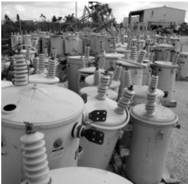
Following the hurricane and due to environmental concerns, the Company established contacts with overseas companies specialising in waste wire, metal and transformer recycling. CUC shipped over 100,000 pounds of scrap aluminium conductor and 350-hurricane damaged transformers to Florida for recycling in 2006.
