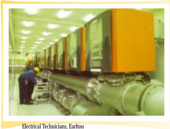
Electrical Technicians, Earlton Bramble and Kurt Hislop, test the relay systems on switchgear equipment in the new 69KV gas-insulated switchgear substation which was completed in summer 2000.
