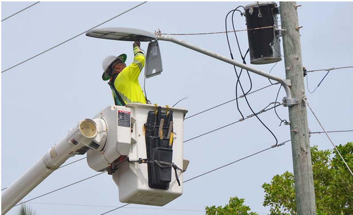
Power Line Technician Chris Bodden installs an LED street light.
